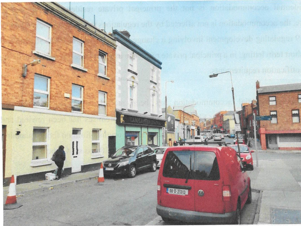
View on Brabazon Street elevation. The Referrers house is on the left, marked by the vertical poles above the parapet erected by the Referrer to enclose a roof garden created at that level since his purchase in 2014.
